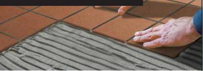
**Metropolitan Ceramics' unglazed quarry tile** Fired in tunnel kilns heated to in excess of 2,000° Fahrenheit for low absorption,added slip resistance, and extreme durability.
