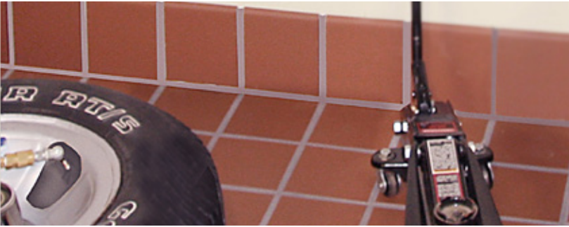
Photo above shows Metropolitan Ceramics Tile used in a service area. The image to the right shows a fulfillment center used by fork lifts and pallet jacks.
